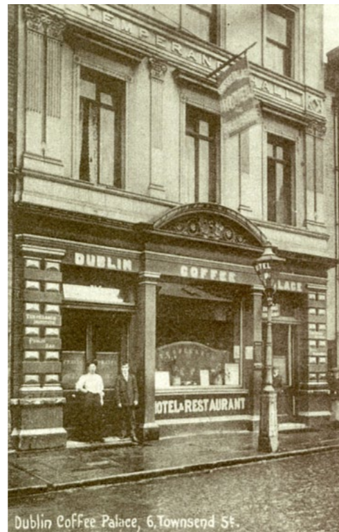
Dublin Coffee Palace, Townsend Street, c. 1900.
